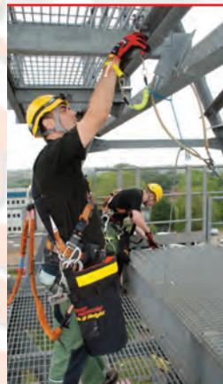
1. Snap-on tools and lanyards are tested and certified. They must not be modified or mixed with products from other sources.
